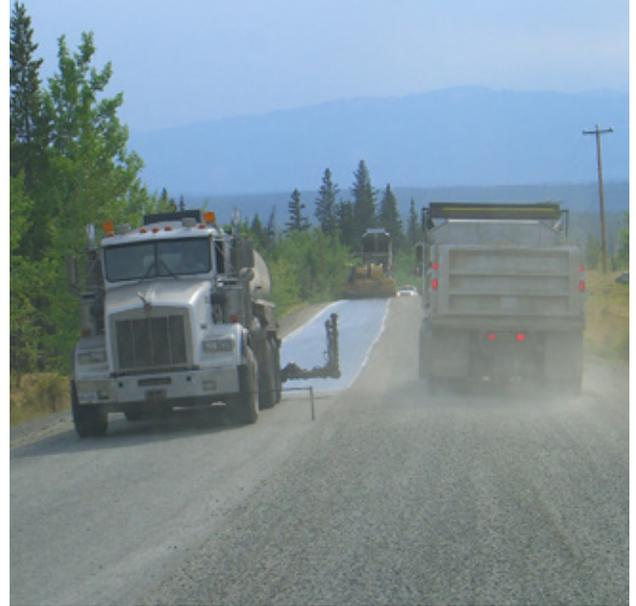
*Seal Coating is the application of a special protective wearing surface to an existing pavement or gravel base.*
