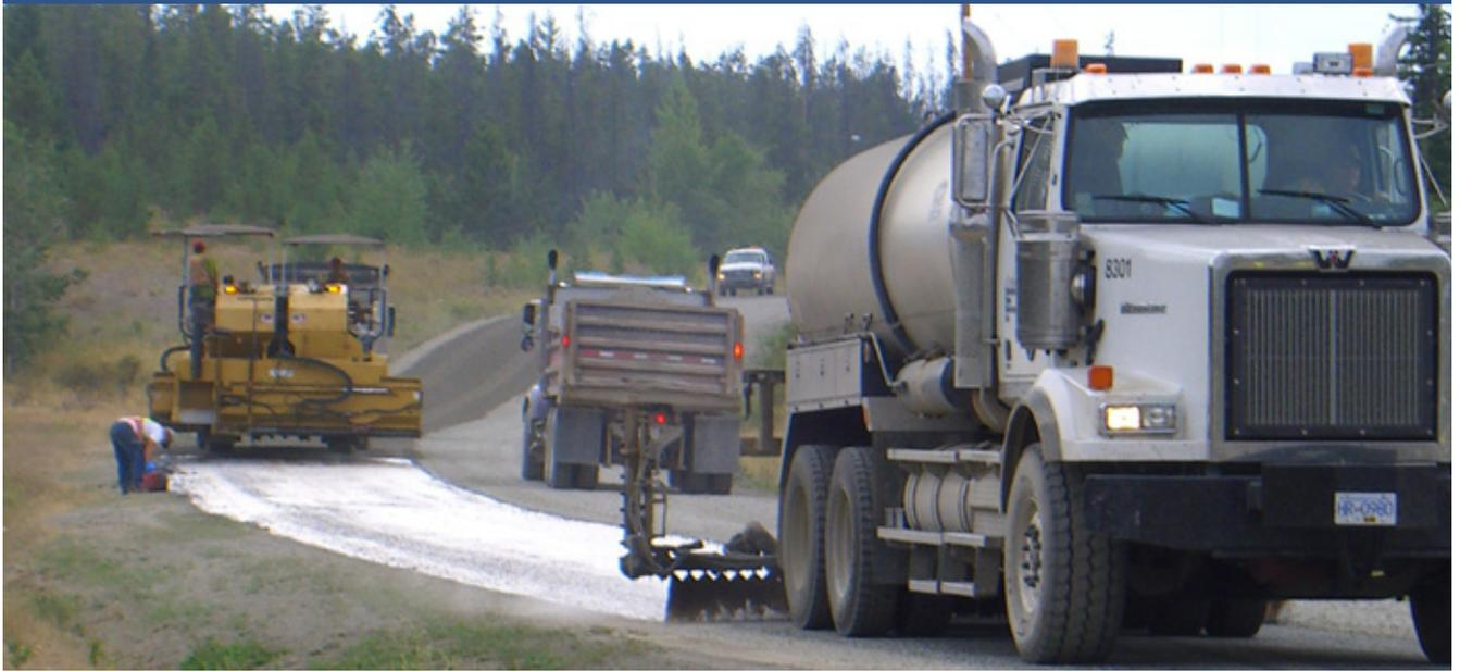
Seal Coating is the application of a special protective wearing surface to an existing pavement or gravel base.
