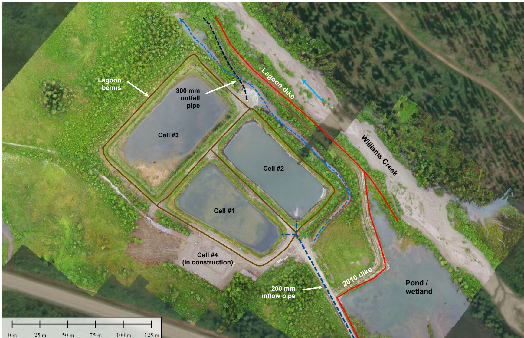
Figure 4-12 BGC June 23, 2025 drone photograph of Barkerville wastewater lagoons.
