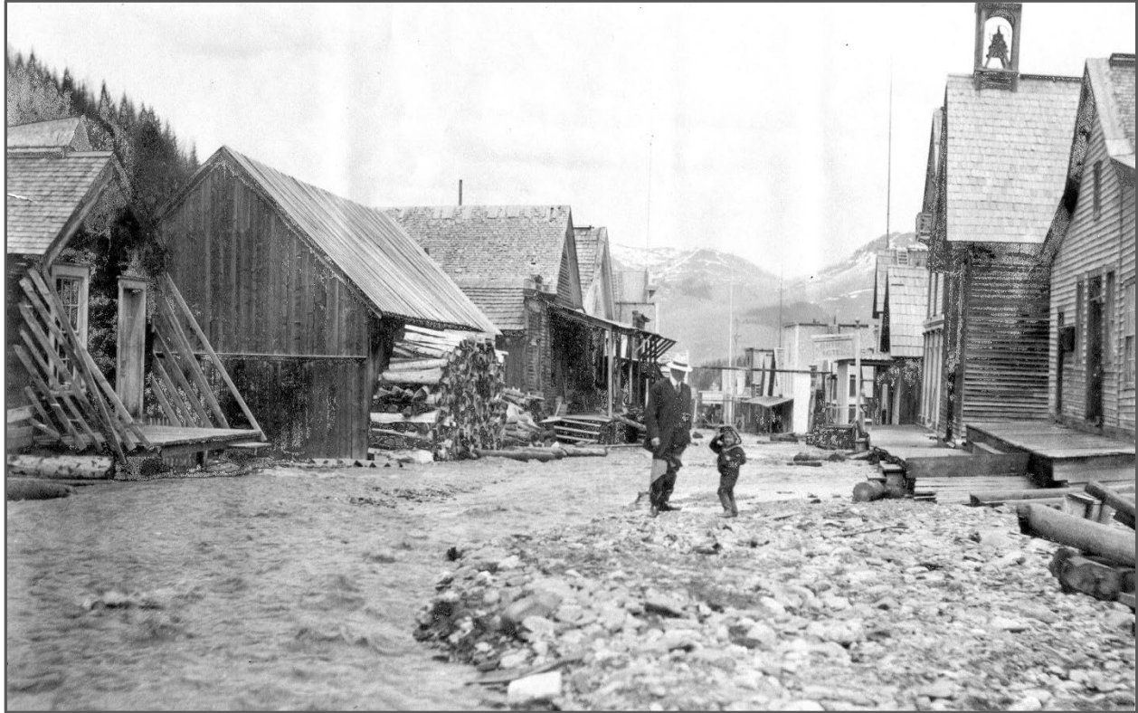
Figure 4-1 Main Street of Barkerville during a flood on June 11, 1911. Barkerville photograph collection, P2767.
