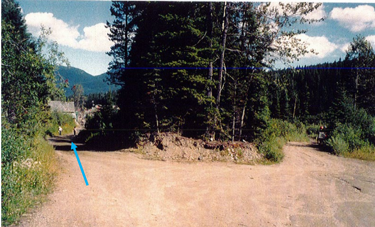
Figure 4-3 View looking north at the south end of the Main Street/service road loop. The blue arrow shows the flow direction that allowed Stouts Gulch overflows to reach the townsite in 1993. Photograph of August 27, 2001 (Galbraith, 2001). McElhanney (2010) recommended that the road be raised in this area for flood control. However, this work was never completed.
