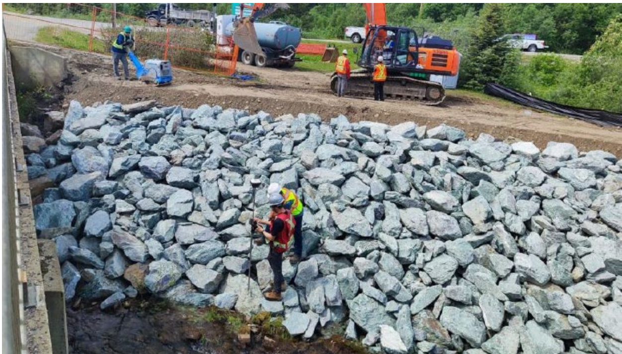
Figure 4-20 Riprap placement on the left (west) bank of Willow River immediately downstream of the Highway 26 bridge. Photo source: Radloff (unknown date).
