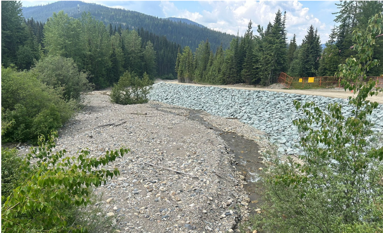
Figure 4-25 Downstream view of Lowhee Creek from the BGM bridge. The Phase 1 and 2a dike is visible on the right bank. BGC photograph of June 22, 2025.
