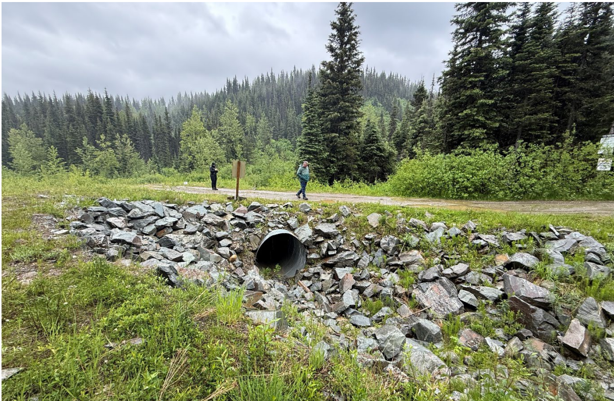
Figure 4-9 Downstream view of Stouts Gulch overflow culvert crossing of Richfield Road. BGC photograph of June 23, 2025.
