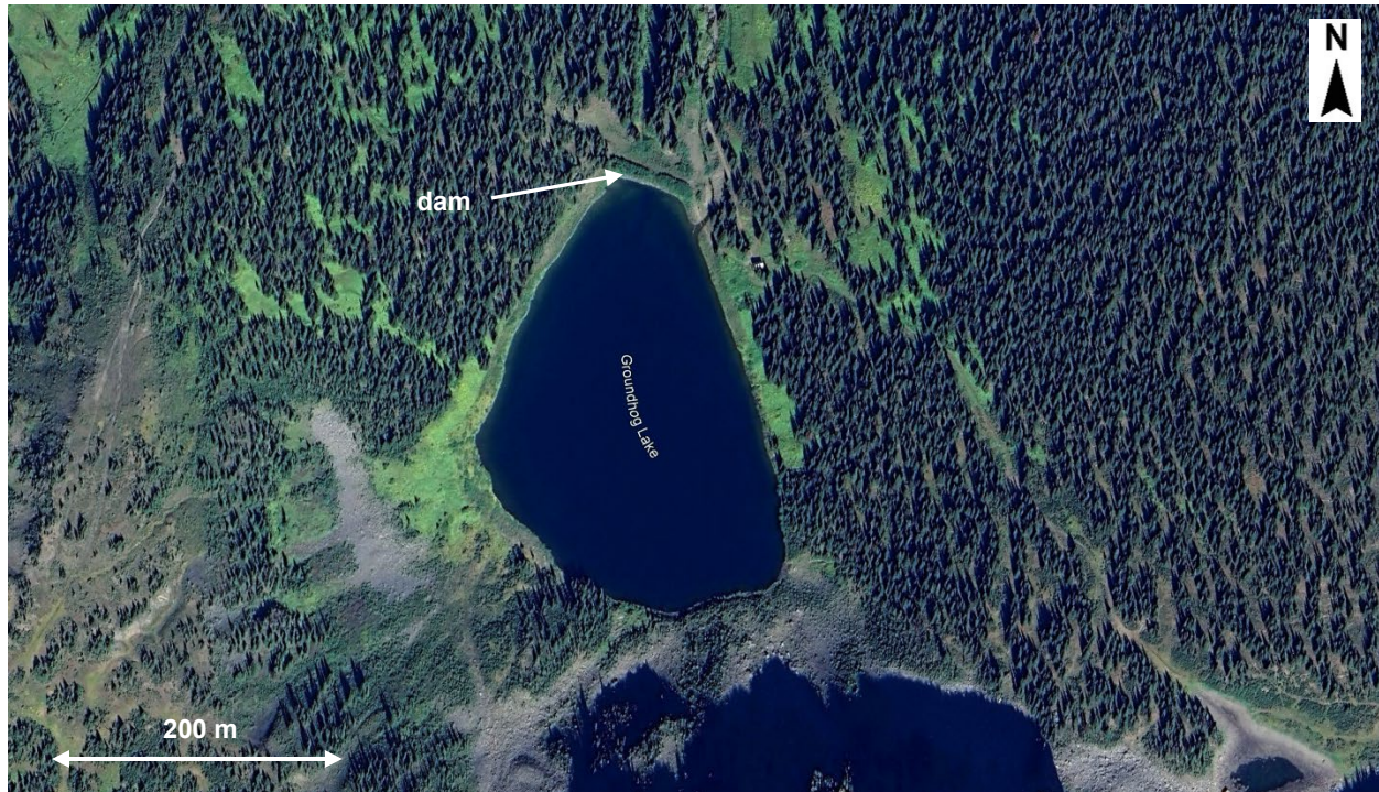
Figure 4-16 Google Earth image (September 3, 2024) of Groundhog Lake.
