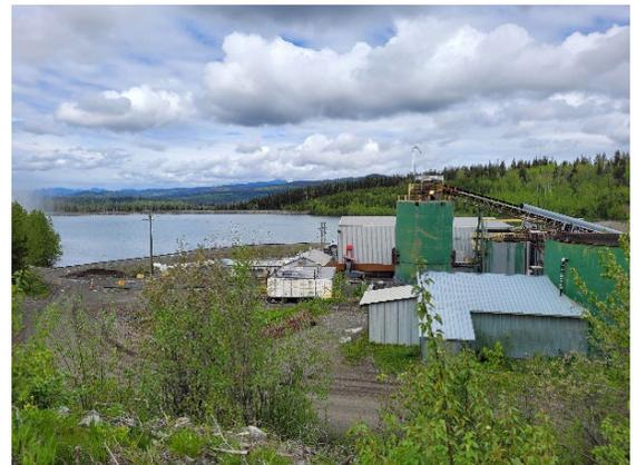
Figure 3: The existing Quesnel River Mill where tailings from Cariboo Gold would be stored
